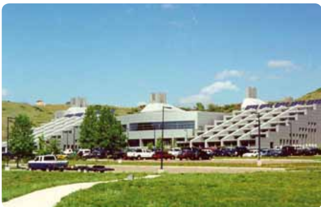
Budova Solar Energy Research Facility institutu NREL
